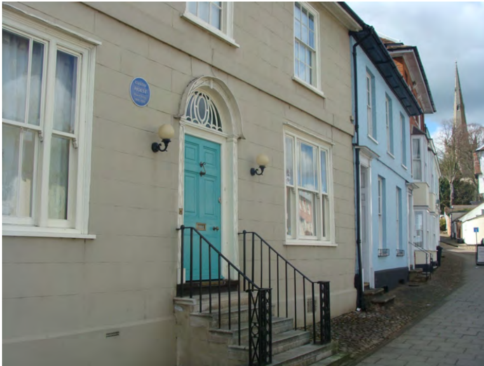
Picture 1.12 Examples of sensitive colour wash to fine listed buildings. It is highly important that this practice continues
