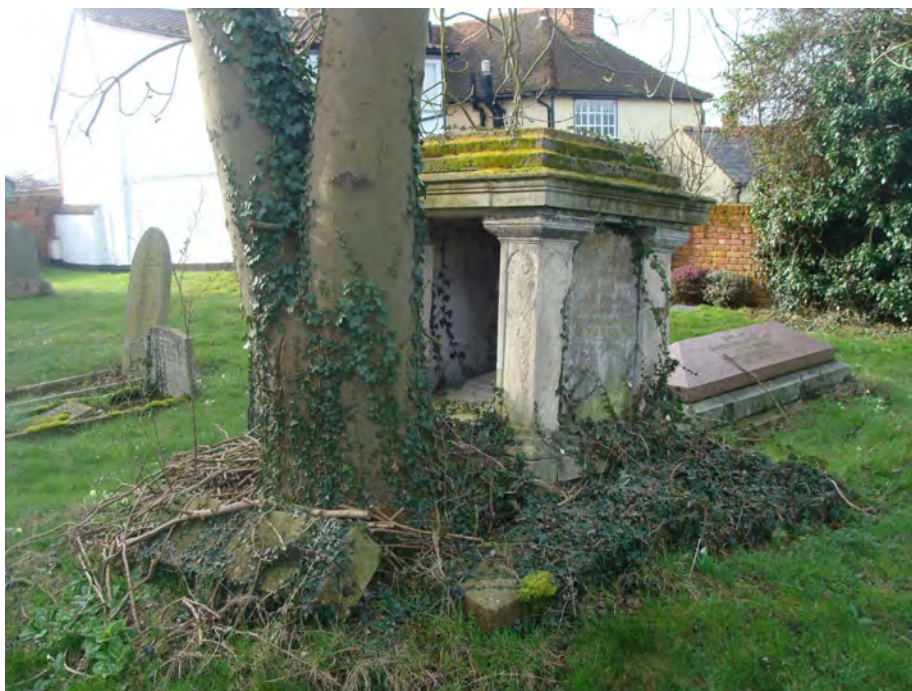
Picture 1.22 Church, some tombs in need of repair; historic graveyard to rear suggested for inclusion in an extended Conservation Area
