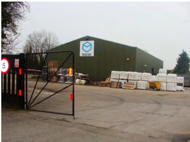
Picture 1.37 Molecular Products site, large scale buildings detract from the quality of the Conservation Area
